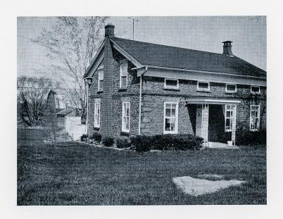
An iron band girdles the house above the first floor windows. This was installed at some previous time, apparently to prevent the walls from bulging too far. 20th century concessions to living are manifest in the front porch and the swimming pool at the rear. The interior is simply and tastefully furnished.
